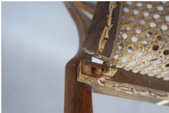
Fig. 5 Detail of broken joint p. right back corner of the frame.
